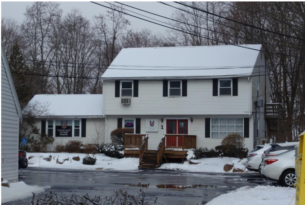
The 1970 commercial building constructed to the north of the Aaron and Lucy Claflin House, on the same parcel.
